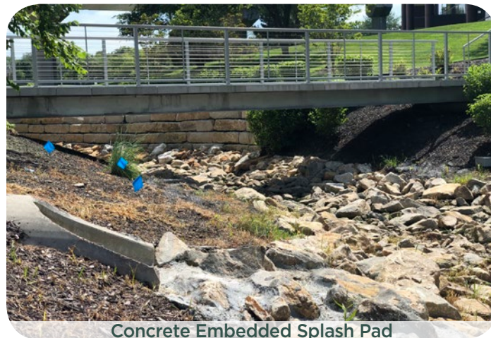
Concrete Embedded Splash Pad
