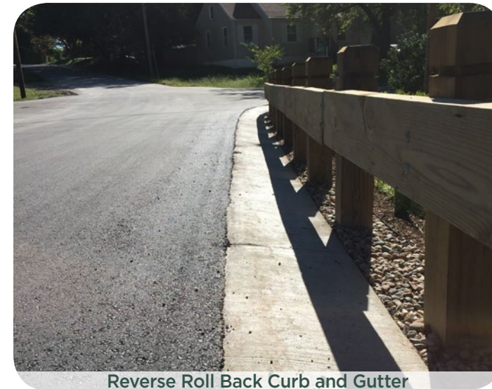
Reverse Roll Back Curb and Gutter
