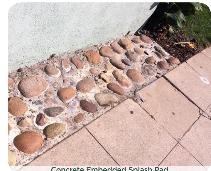
Concrete Embedded Splash Pad
