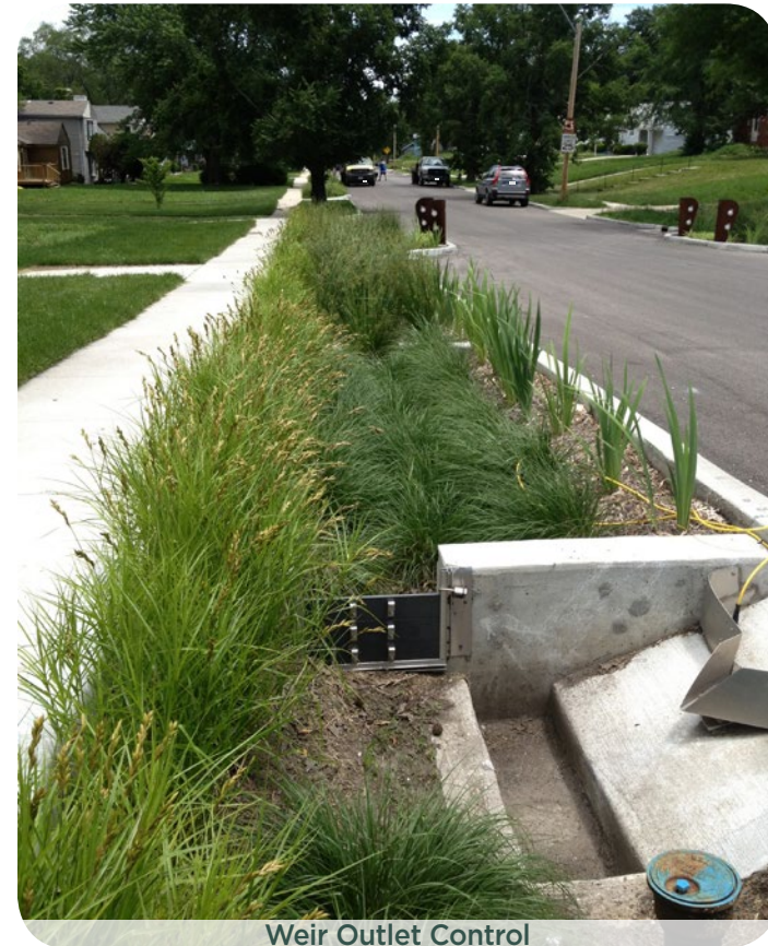
Weir Outlet Control
