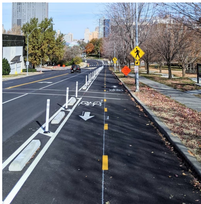
Figure 81: Gillham Road Cycle Track
