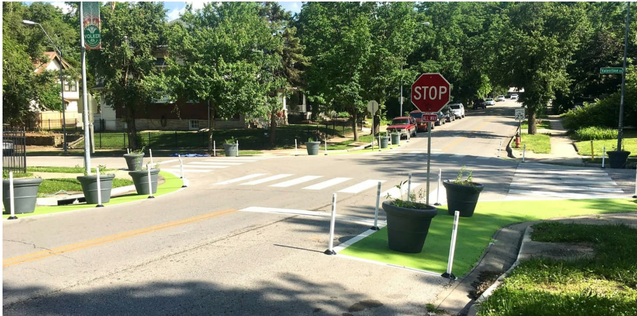
Figure 77: All way stop and traffic calming installation at Wyoming St and Valentine Rd (Image source: Street Smarts Design + Build)
