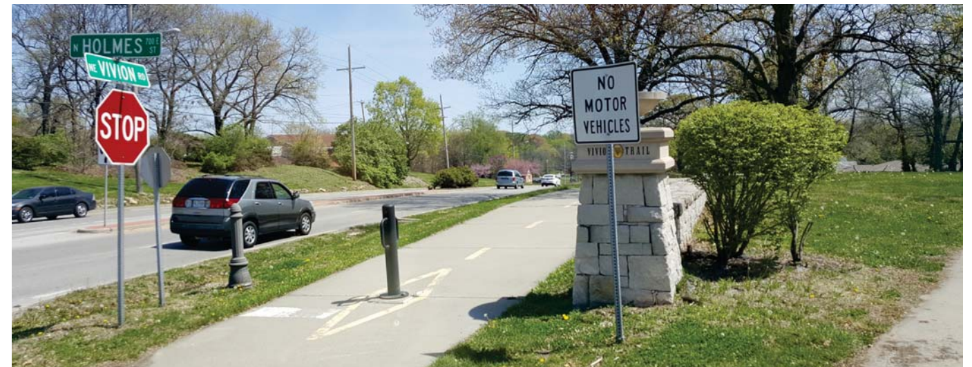
The top image demonstrates the widespread lack of sidewalks along the corridor, specifically within commercial nodes. The bottom image shows the extent of the bike network along Vivion Road: the Vivion Trail.
