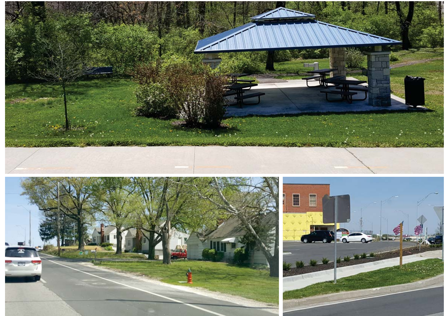
The top image shows a well-maintained sidewalk; the sidewalks that do exist along Vivion Road are generally in good condition. The bottom left image shows the lack of curbs and gutters, though the bottom right image depicts a recent curb and gutter installation at Antioch Road, as well as other infrastructure improvements.
