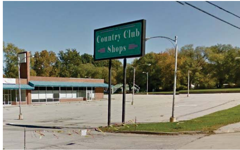
The top image shows the widespread lack of and poorly maintained landscaping along Vivion Road, specifically within the public right-of-way. The bottom image demonstrates the all too frequent commercial parking lots that front the roadway with no interior landscaping and minimal screening. The bottom image also shows an outdated pylon sign. While not a frequent occurrence, such signs date the corridor and may provide inaccurate information.
