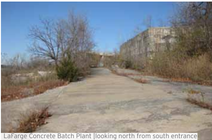
LaFarge Concrete Batch Plant | looking north from south entrance
