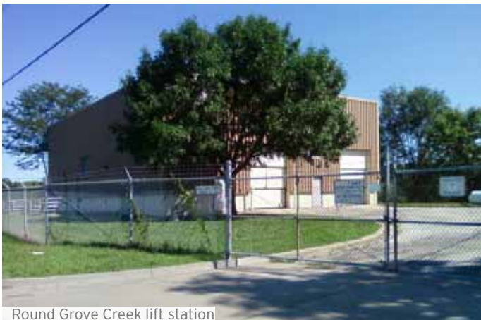
Round Grove Creek lift station
