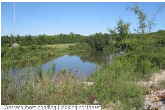
Western-most ponding | looking northeast
