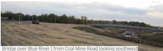
Bridge over Blue River | from Coal Mine Road looking southwest
