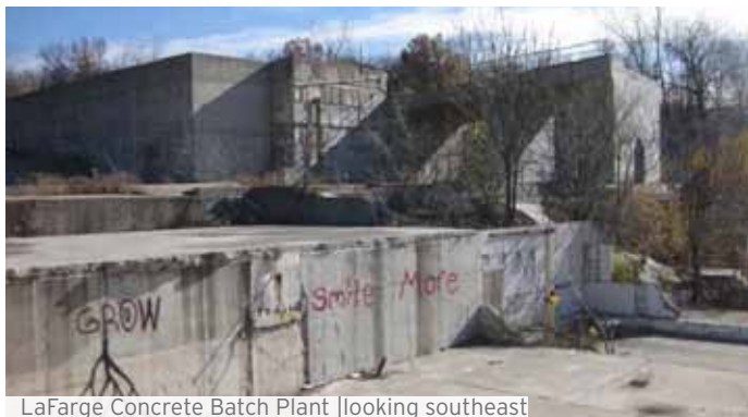
LaFarge Concrete Batch Plant |looking southeast
