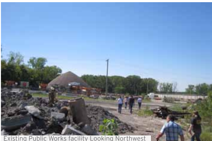
Existing Public Works facility Looking Northwest
