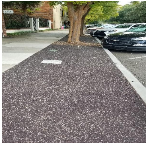
Figure 4: Existing curb with existing sidewalk
