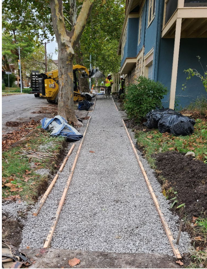
Figure 10. Rubberway section prior to installation
