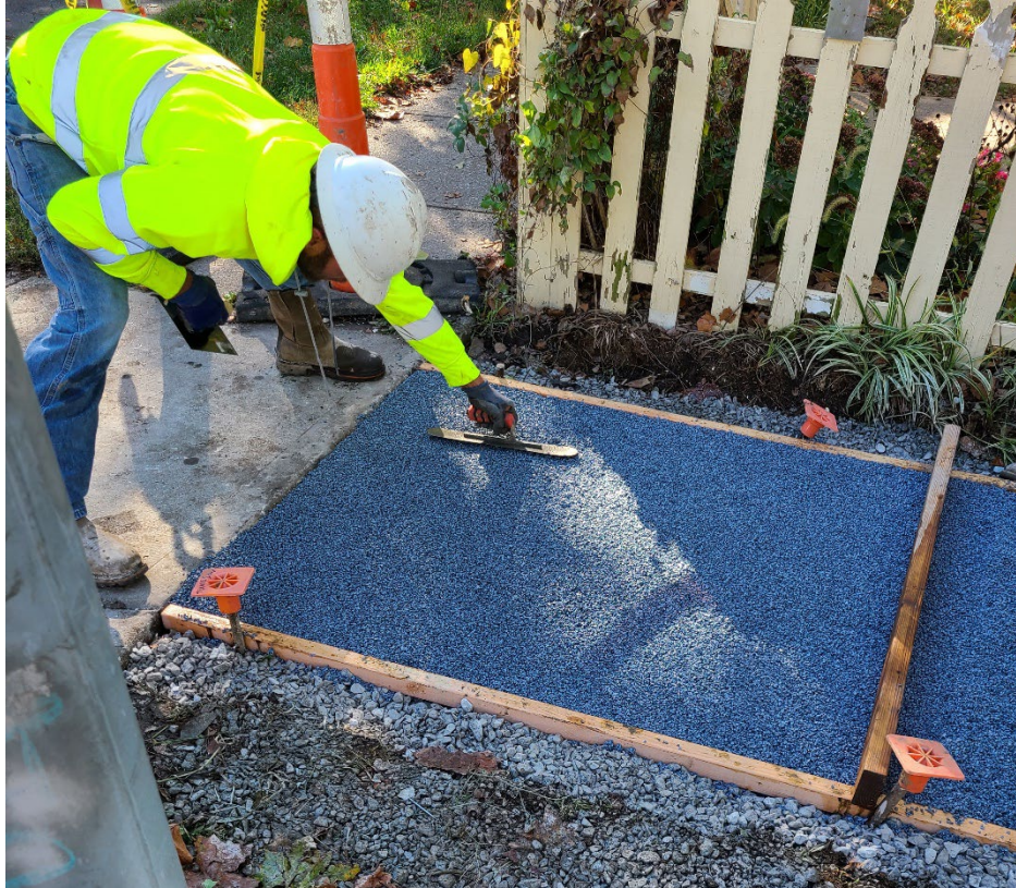
Figure 13. Finishing Rubberway section with hand trowel
