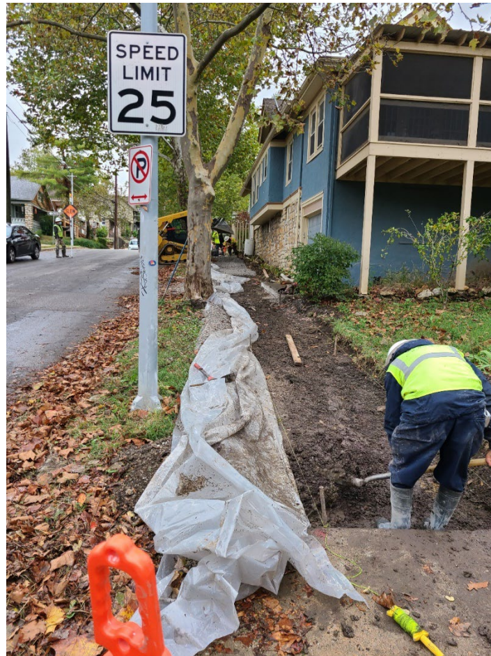
Figure 7. Rubberway section looking east prior to installation of aggregate base materials
