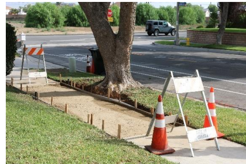
Figure 2: Temporary wood forms
