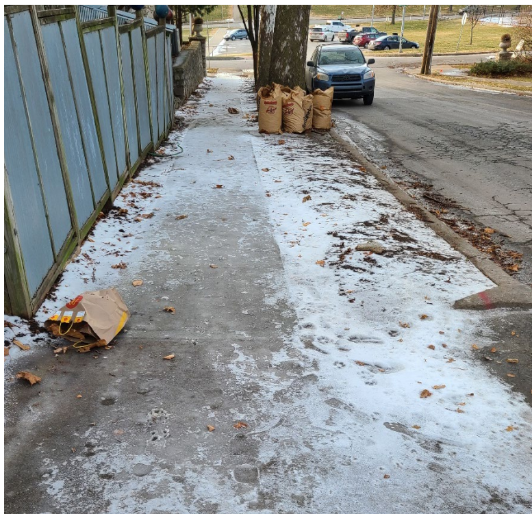
Figure 21. Concrete research section unplowed during winter
