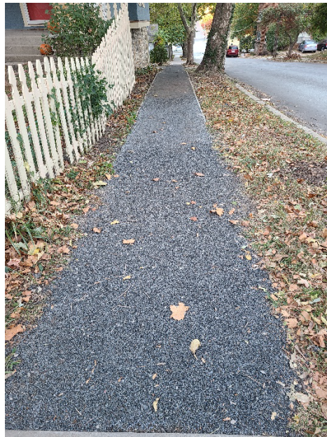
Figure 20. Current state of the bad Rubberway section (Oct 2022)
