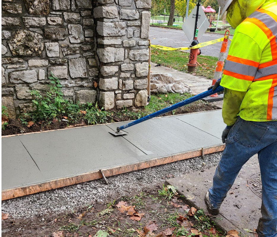
Figure 16. Hand tooling joints in the research concrete section
