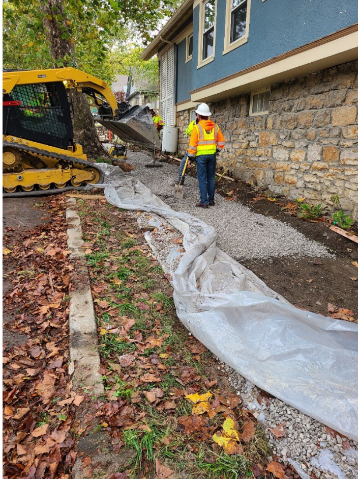
Figure 9. Rubberway section during aggregate base installation
