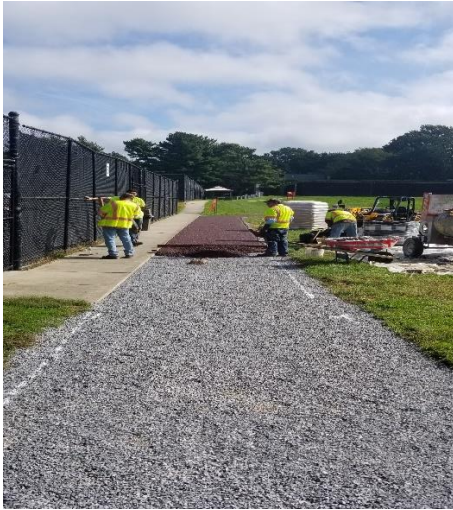
Figure 3: Line the base rock if forms are not used
