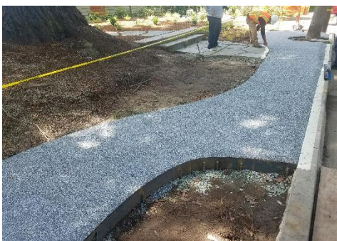
Figure 1: Concrete curb with Steel Edging
