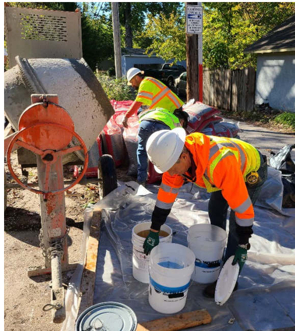
Figure 11. Day 1 Rubberway mixing
