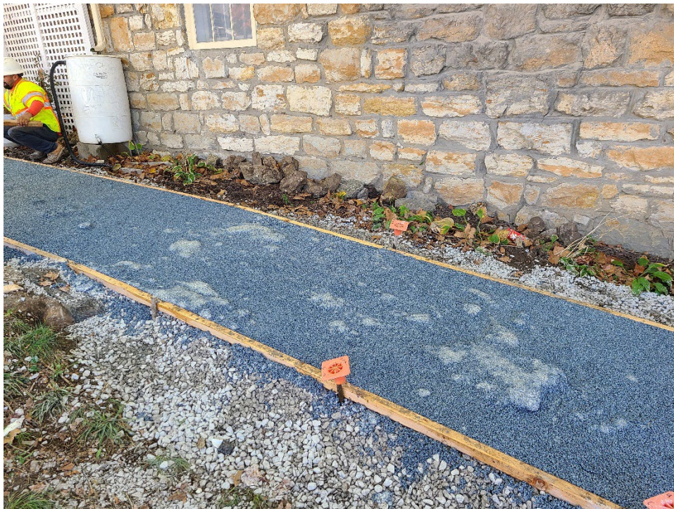
Figure 15. Continued bubbles forming prompting a halt of day 1 placement
