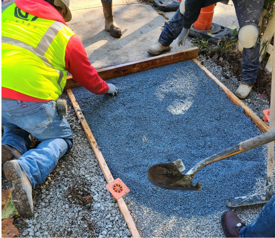
Figure 12. Initial installation of Rubberway section
