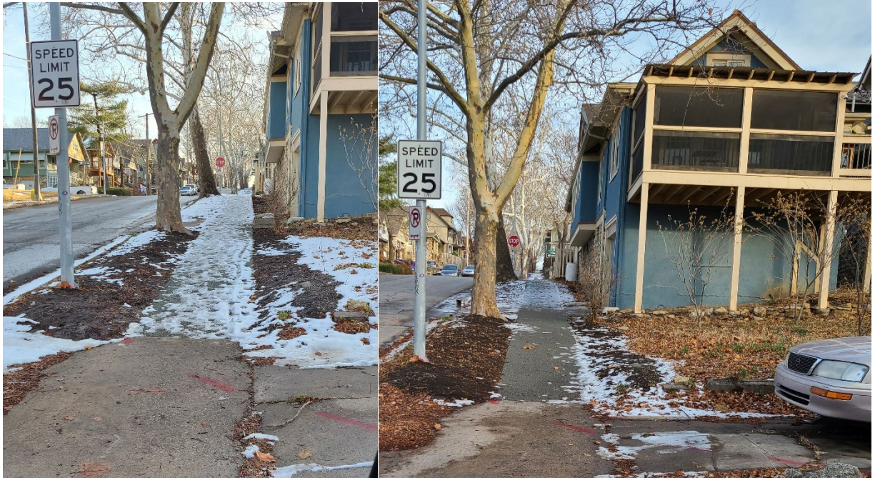
Figure 19. Unplowed Rubberway section where section exposed to sunlight melted and shaded did not
