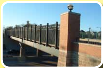
Distinctive bridge structures
