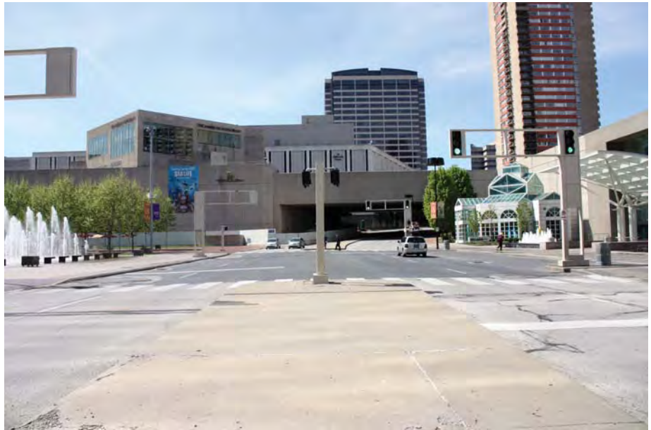
Existing view of plaza / vehicular space within Crown Center. The concrete median should be removed.
