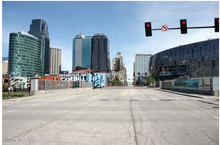
Image Looking North across I-670 Bridge
