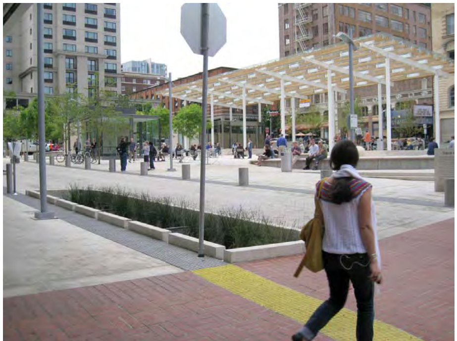
Example project that showcases a curbsless plaza and vehicular path with stormwater best management practice for stormwater filtration.
