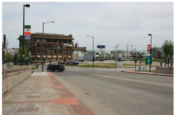
View existing I-70 bridge
