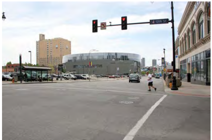
Image looking at 13th Street Parking
