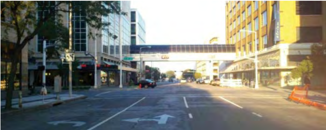
Design of Bi-directional Bike Facility in Lincoln, Nebraska (Demonstration Project Opens in 2012)
