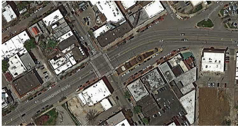
Existing Conditions Aerial Photograph
