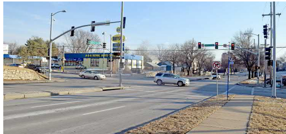
Bad Transit Facilities
