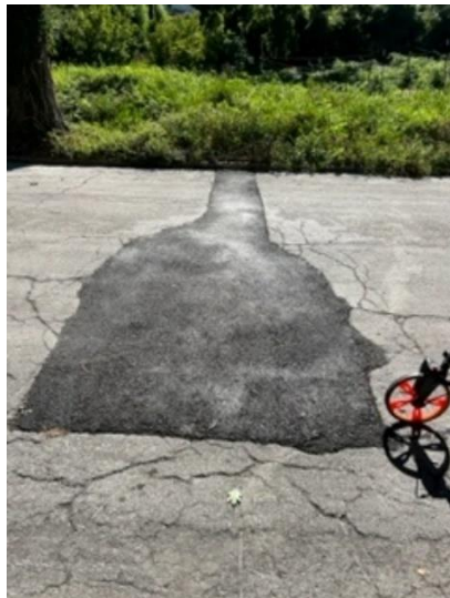
Exhibit 6. Older Streets - Street Excavations Not Restored to Standard
