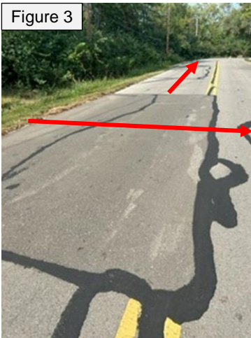
Figure 3. Width of repaving is not to required 2 lanes and length of repaving is not to required block face or 250' maximum.
