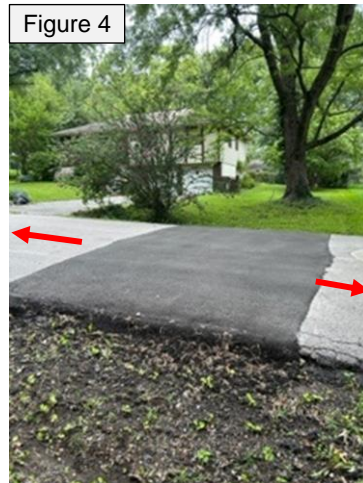
Figure 4. Length of repaving is not to required block face or 250' maximum.
