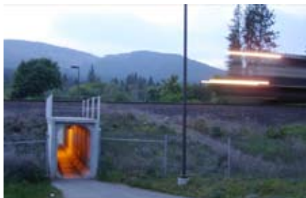
Trail underpass with railroad buffer
