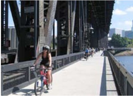
Shared-use trail bridge in Portland, OR
