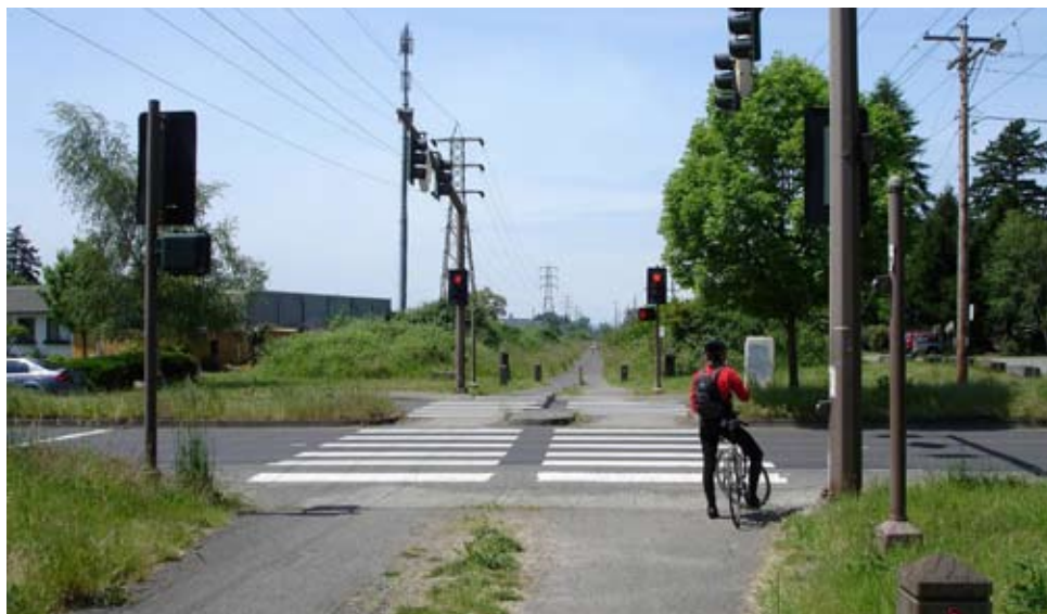
Signalized crossing with continental striping
