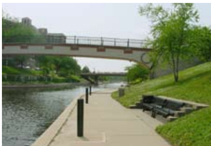
Existing Brush Creek Trail
