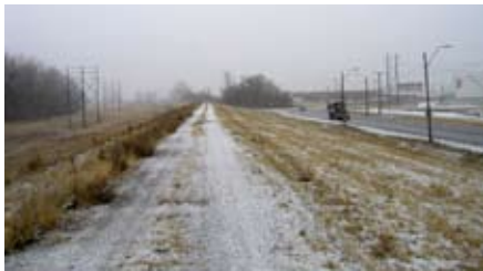
Levee Trail – existing levee conditions
