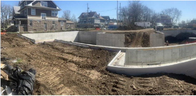
Backfilled - Southeast Wall
