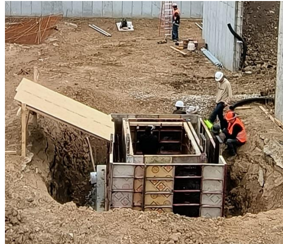
Elevator forms ready for concrete.
