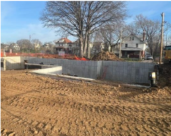
Backfilled - North at middle to northeast
