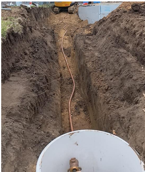
Water Supply Line
