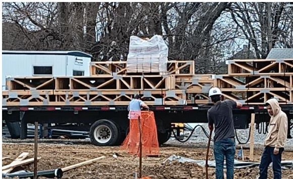
Lumber – first level and floor trusses
