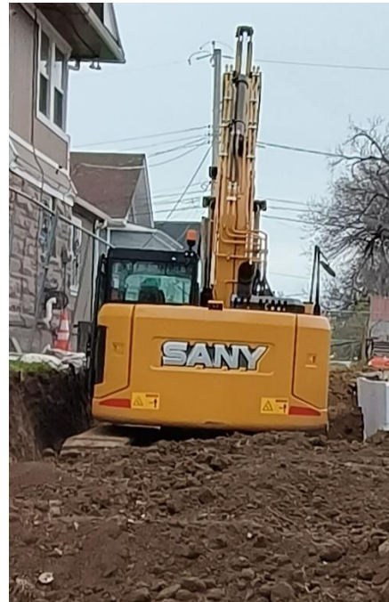
Backfilling – eastern wall
