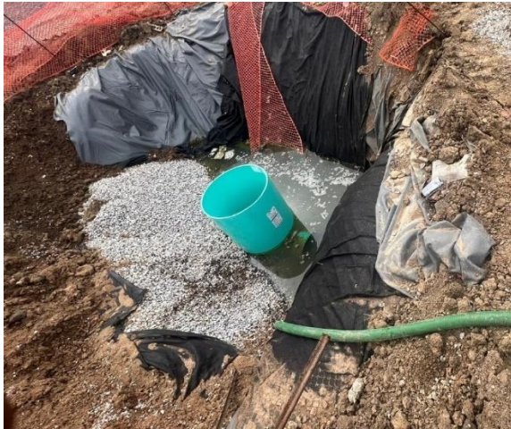
Drainpipe installation
