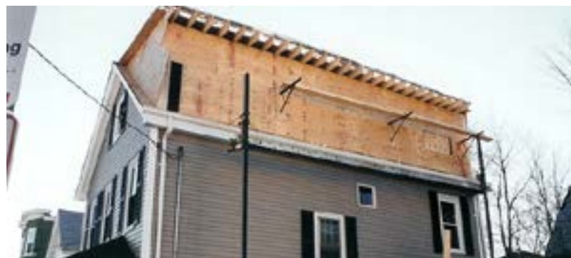
NOT RECOMMENDED The scale and style of the dormer is not compatible and with the existing building.
