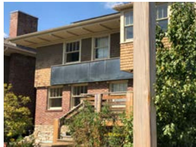
Solar Collectors on House in Rockhill Kansas City 16
