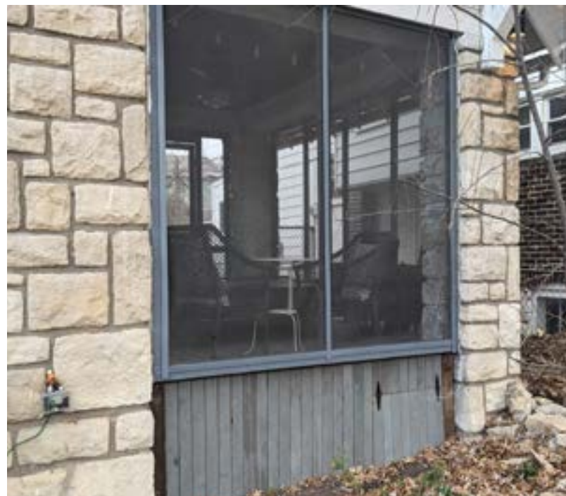
Porch reused as deck skirt. Credit: Amanda Wilson 23
