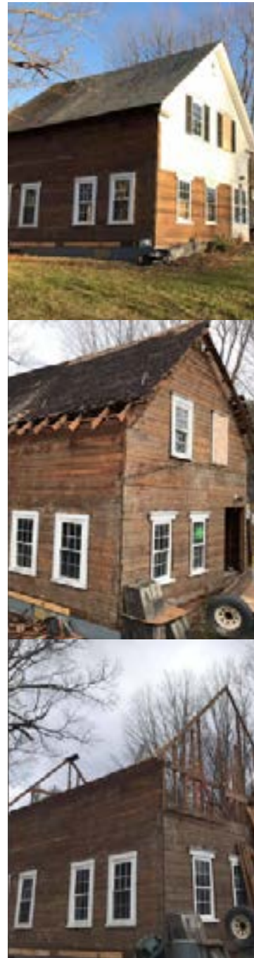
Deconstruction Progress Site 21 Credit: Deconstruction Works
