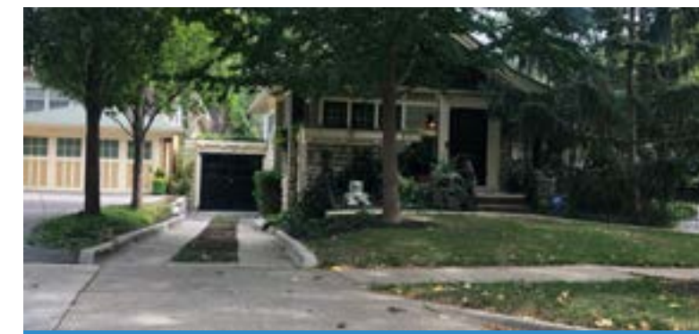
RECOMMENDED The strip paving minimized the impact to the natural landscape.
