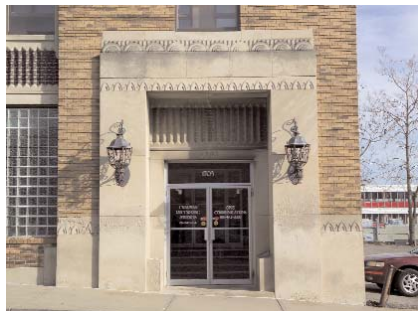
Facade lighting that complements the architectural character of buildings.
