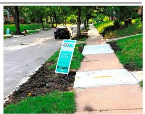
the entire depth and width of the concrete slab to reduce cracks and allow a clean break if old and new slabs need to be separated. For example, on one block, expansion joints were not installed at 35 locations where old and new concrete met.
