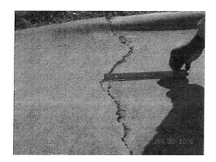
2. Any driveway that differs vertically by more than 1 inch either above or below the sidewalk shall be replaced. (by more than ½ inch within the downtown loop area.)\*
