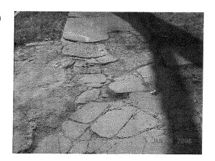
5. Any square that is upheaved or depressed, thereby causing an abrupt change in grade beyond specification shall be replaced.
