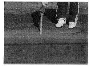
2. Any curb having a gutter section of 4 inches or more below the street surface measured at the edge of pavement shall be replaced to the nearest joints.
