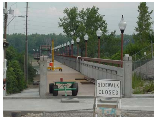
Pedestrian Bridge Under Construction
