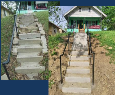
Stair and Handrail Replacement
