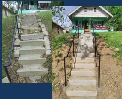
Stair and Handrail Replacement
