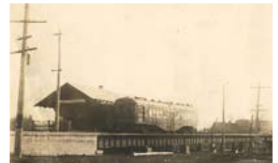
Past active rail line.
