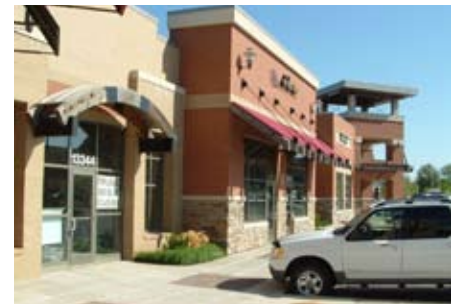
Architectural store front
