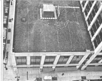
Support: A building across from the Henry has a roof planted with greenery to insulate and to reduce runoff.
