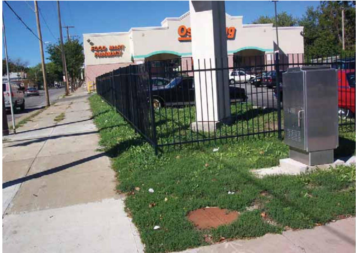
Parking lot screened with a black, wrought iron fence. No street trees present along Troost Avenue to buffer pedestrians from the roadway.
