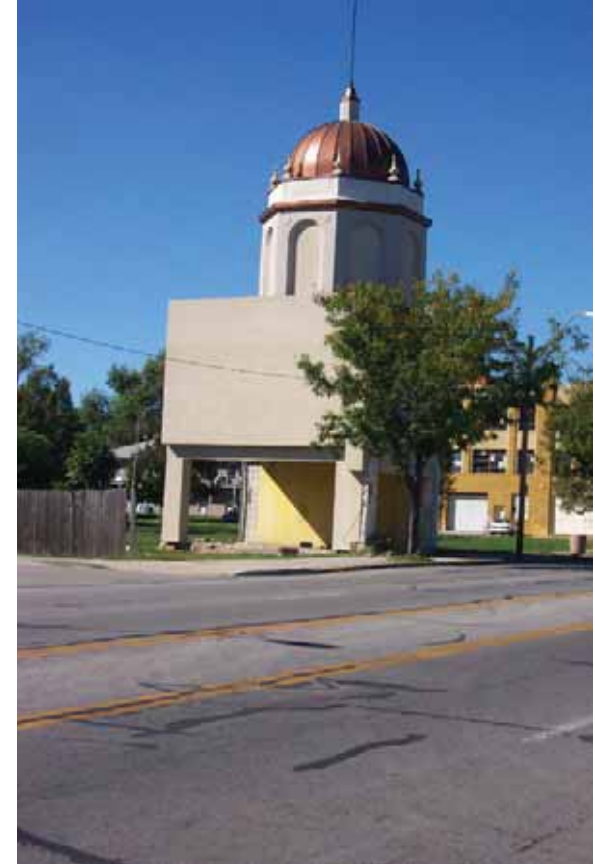
Single building remnants remaining on street.
