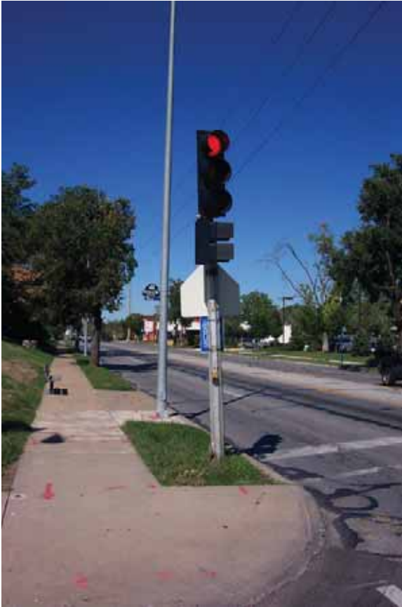
Traffic signal without pedestrian signals.
