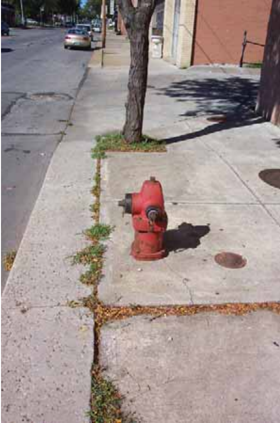
Fire hydrant and street tree. Sidewalk condition is unsightly.
