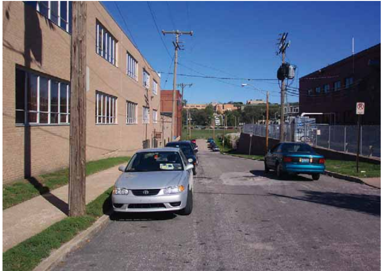
View east down 48th Street to Paseo. The side street character is utilitarian.
