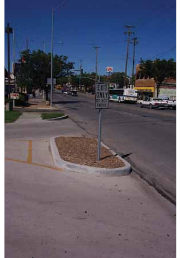
Existing signage and curb cut.
