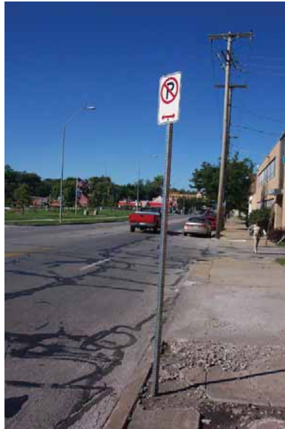
Regulation signage and deteriorating sidewalk.
