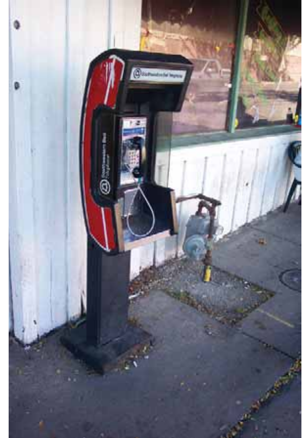
Pay phone with numerous cigarette butts. Sidewalk around gas meter is missing.
