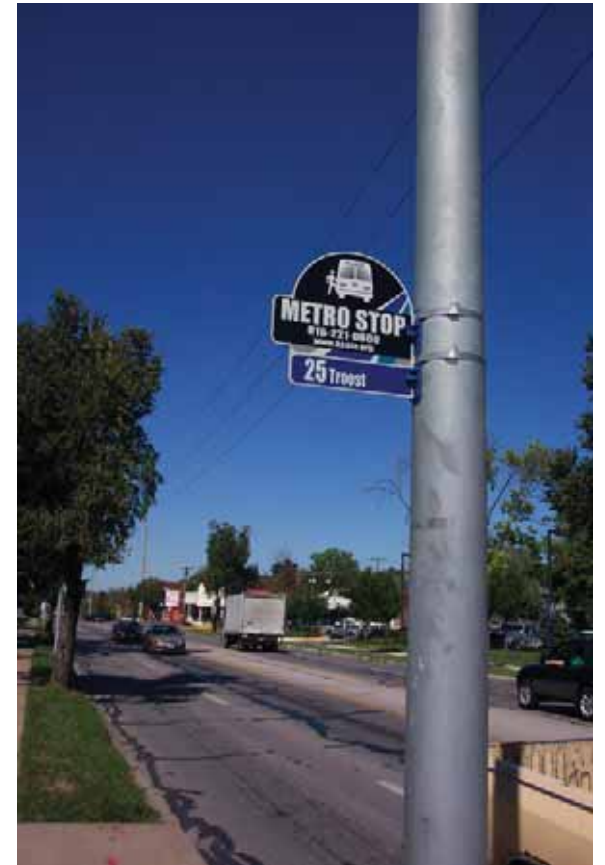
Transit stop signage mounted to existing utility pole.
