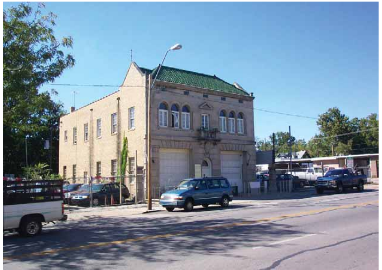
Surface parking is secured with a utilitarian chain link fence. Lone building is present with “gaps” on either side.
