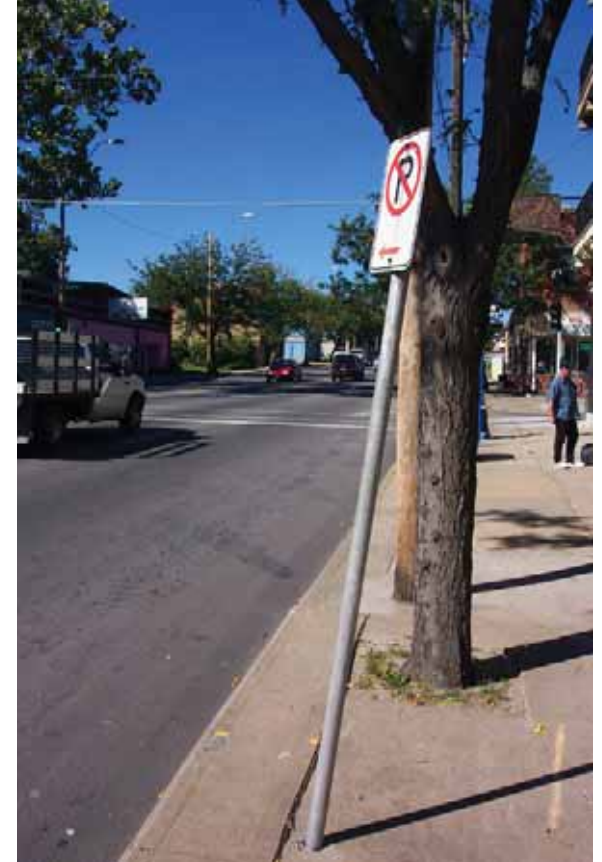
Existing signage mounted on a round, galvanized post. Street tree with a minimal water and air infiltration zone.
