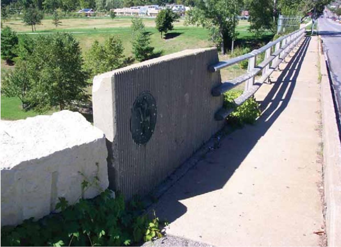
Existing bridge guard rail and pedestrian walk.
