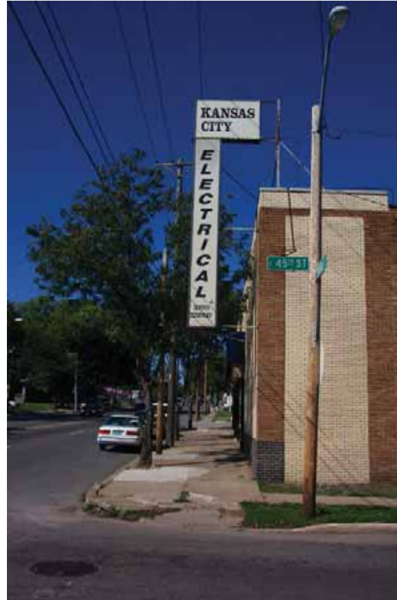
Storefront signage. Existing pedestrian walks are deteriorating and pose a safety and accessibility problem.
