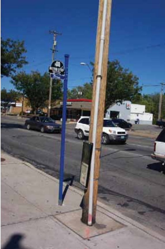
Transit stop signage with map attached to utility pole. No consistency exists between materials.
