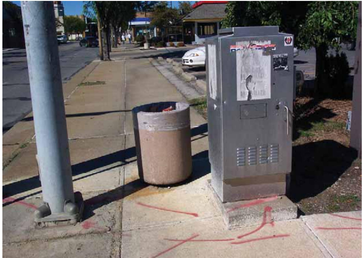
Utility box and trash receptacle placement restrict pedestrian movement.
