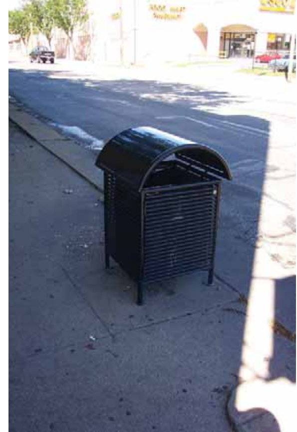
Broken glass remains at the trash receptacle.
