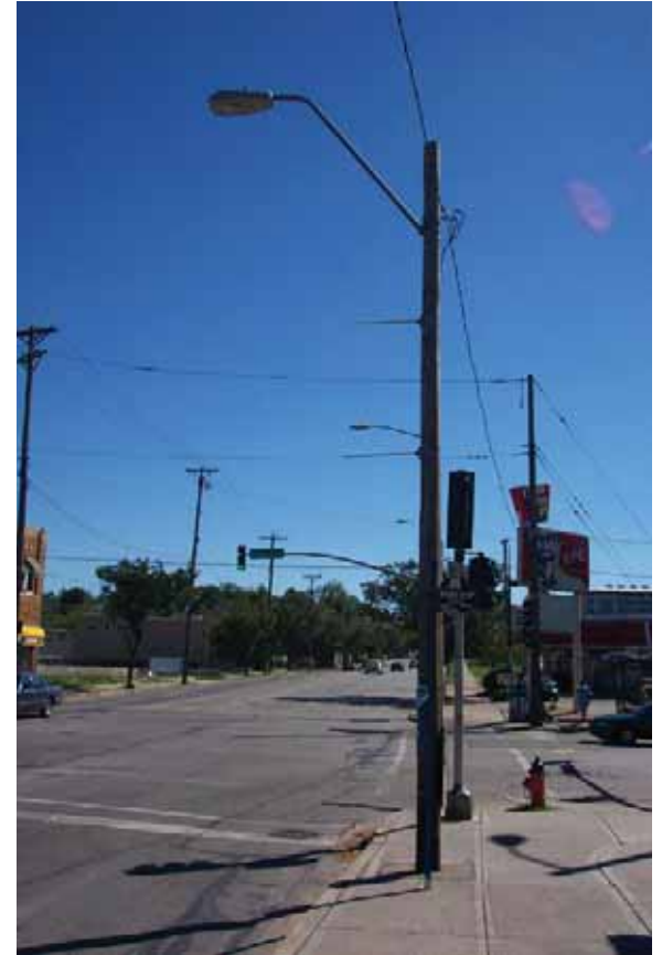
Existing wood streetlight and metal traffic signal. Intersection is stark and unwelcoming.
